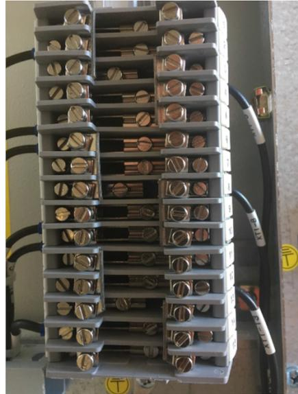
CT terminal block with the links on 3, 8, and 13 open. This is the correct operating position.
