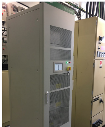
Pictured left, the 300kVAR ASVG unit installed in the Cheese Packing Switch Room
