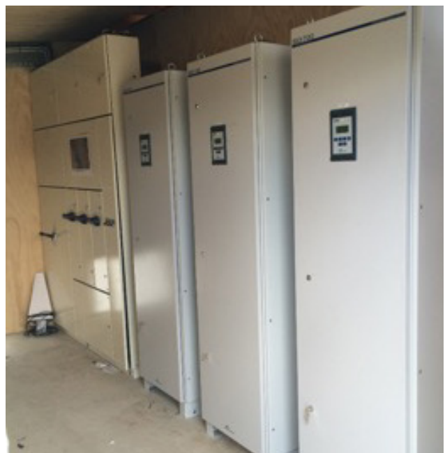
The 73 million litre storage lake and some of the SD700 “Active Front End” at Terrace Water, Central Otago.
