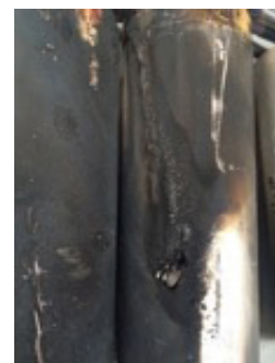
A capacitor that has “burst” through the side of the can and released pressurised gas that has caught fire
