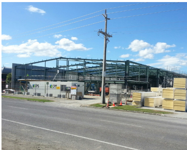
The new plant under construction
